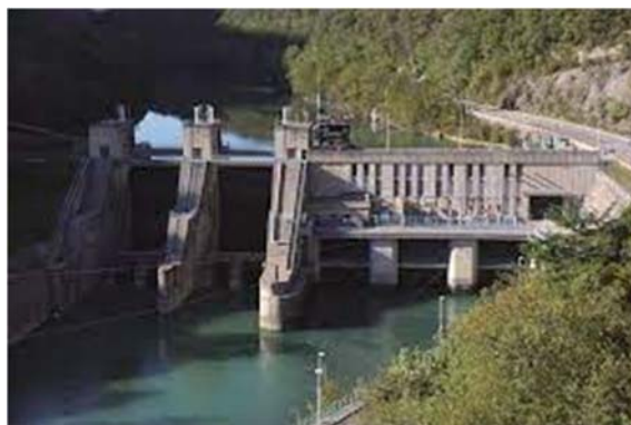
Figure 24. Solkan Dam on the Isonzo/Soča river. Source: AAWA, 2021.
