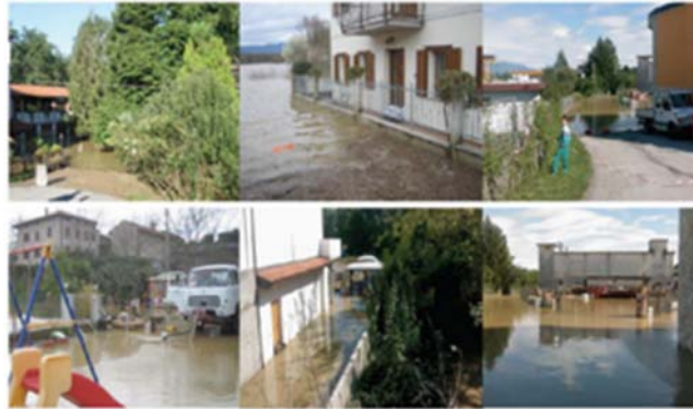
Figure 26. Flooding in the Slovenian Part of the Vipava/Vipacco River in occasion of the flood of 2009 and 2010. Source: AAWA, 2021.
